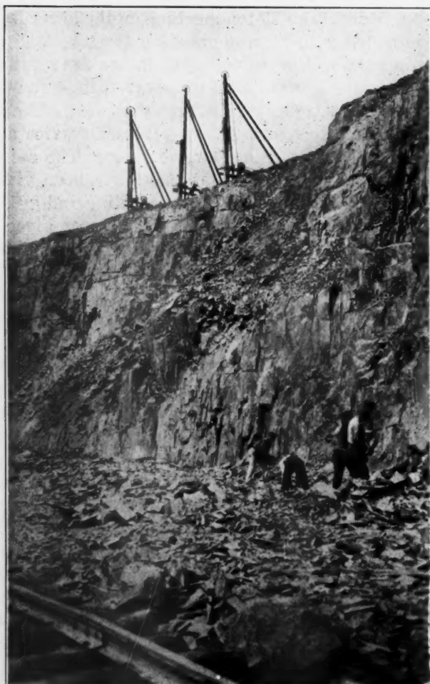
Drills at Work on Top of Bench
